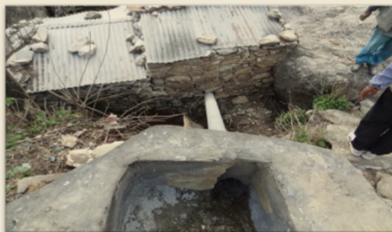
Water Intake- after Modernization
