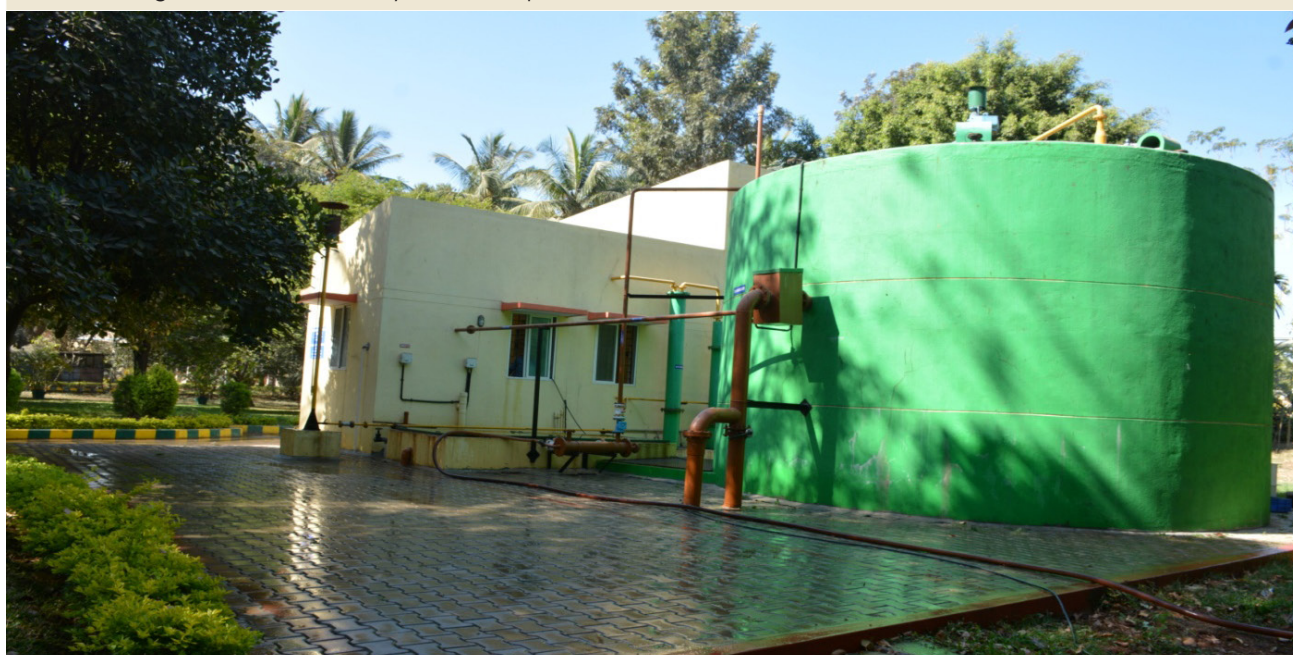
Image 15 Bio-Methanation plant for Handling of Food Waste
