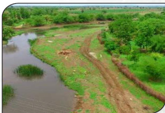
Widening & De-silting of Seasonal Nallah (1 km)
