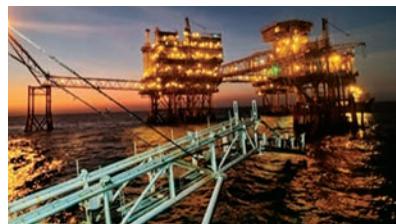
Start of pipelaying from Panna Process-A (PPA) platform
