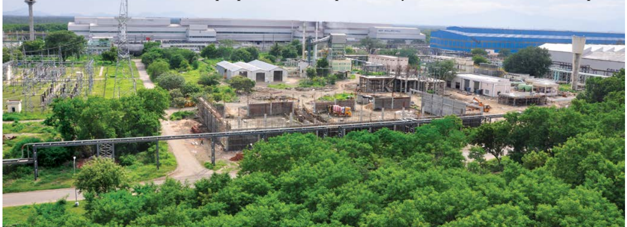
View of Green SAIL Steel Plant at Salem.
