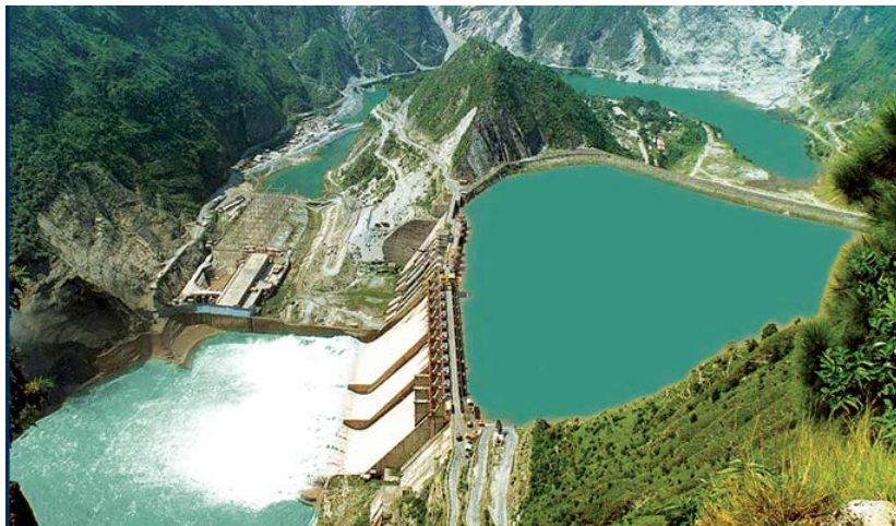
690 MW Salal Power Station (Jammu & Kashmir) - Concrete Dam
