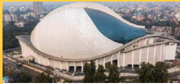
DHANA DHANAYE AUDITORIUM AT KOLKATA
