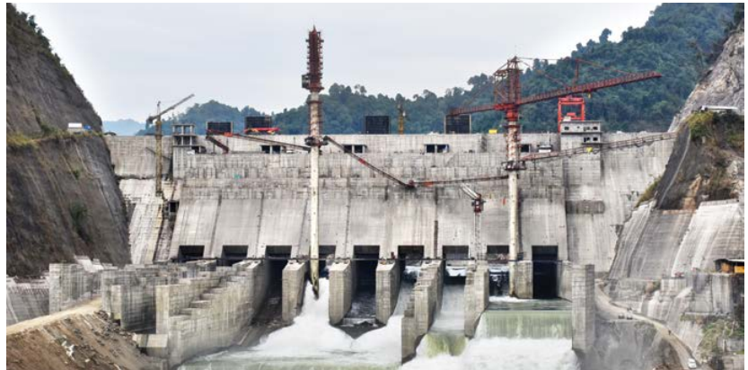
2000 MW Subansiri Lower HE Project (Assam/ Arunachal Pradesh) – Dam
