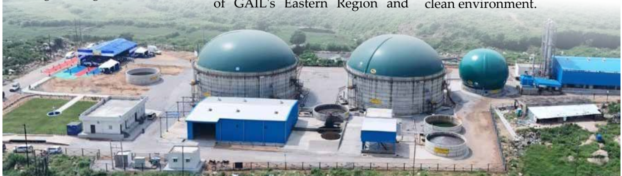
GAIL (India) Limited's Compressed Bio Gas (CBG) plant in Ranchi, Jharkhand.
